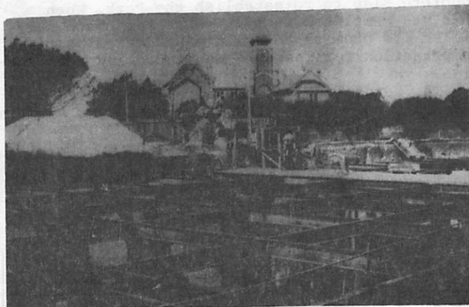
Excavation for Gladstone Park Reservoir : c1917
