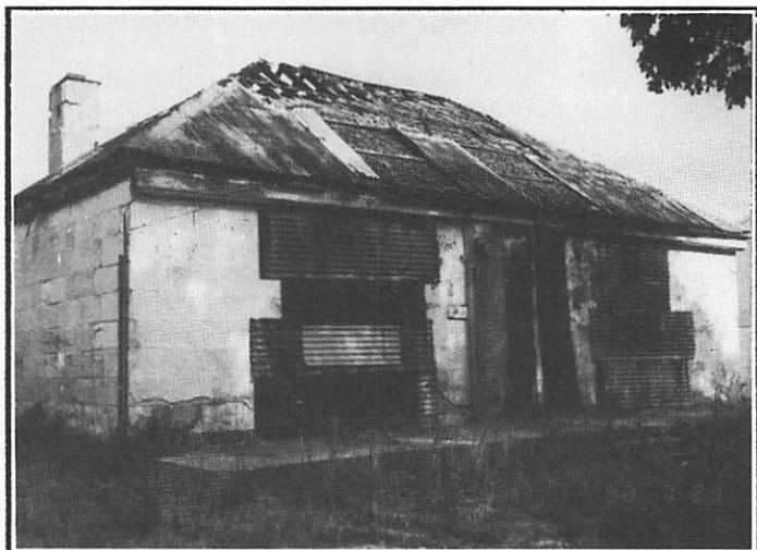
Clontarf cottage before restoration
