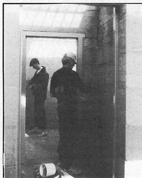
Further pictures of the Watch House restoration. Far left: Ian Smale working on the Kitchen. Left: Kel and Jason Munyard repointing cell walls.
