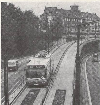
The city of Essen has met the increasing challenge individual transport poses to public transport. The first track-guided bus operation commenced in 1980. Since 1988, these buses have shared the city tram tunnel to avoid city centre traffic chaos. Passengers enjoy a smooth trip to the city without interruptions, past congestions.
