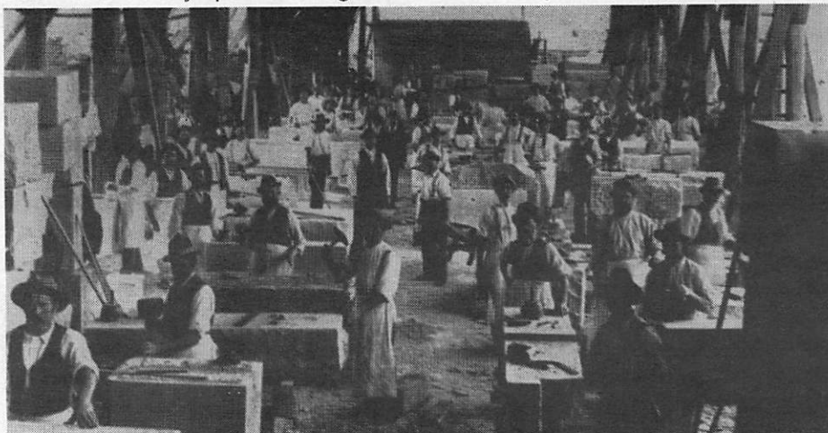
Stonemasons preparing foundations
