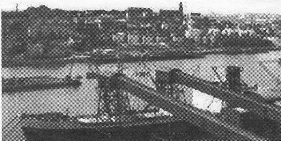
Esso Oil Storage White Bay 1967
