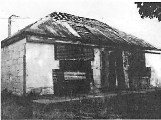
Clontarf Cottage before restoration
