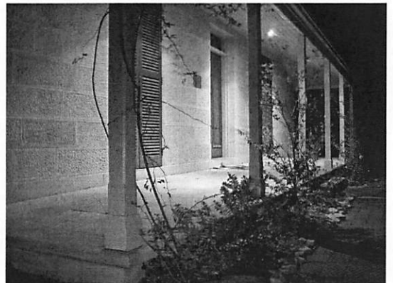
Clontarf Cottage after restoration
