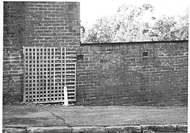
The Cameron Street wall
