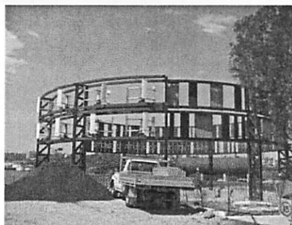
New, Tank 101, under construction
