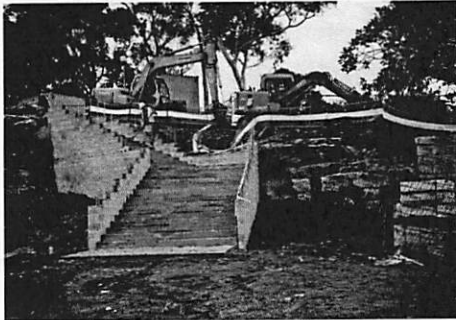
Peacock Pt steps, construction
