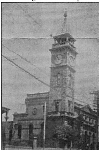
better view of the side of the iconic 1886 James Barnett Post Office tower.
