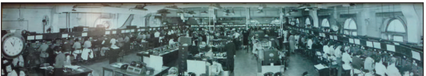
A 1956 photo of the Sydney GPO Interstate Telephone Exchange
