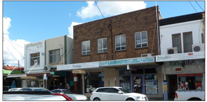
The view before the September fire, showing modern repairs to storm damaged heritage buildings.
