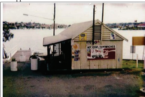
Above: Waiting room/kiosk date unknown most likely 1970s/80s Leichhardt Council files.
