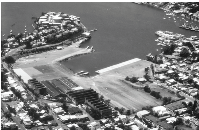
An aerial view of Mort Bay during the construction of the ANL Container Terminal in 1968.
