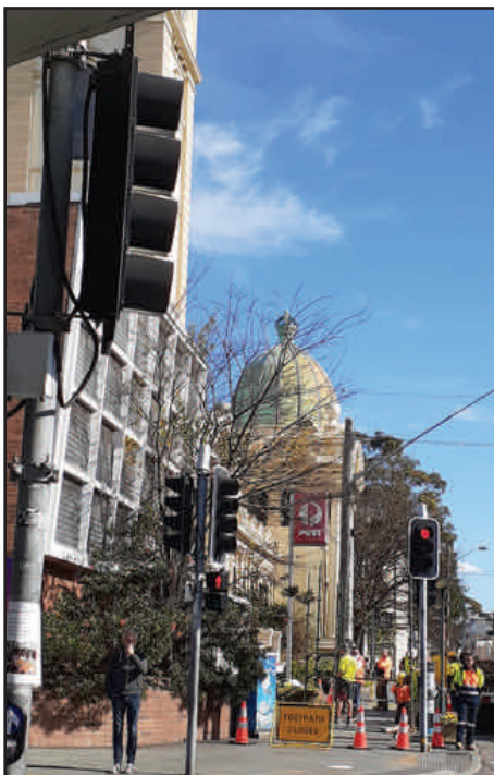
Start of demolition early August 2019
