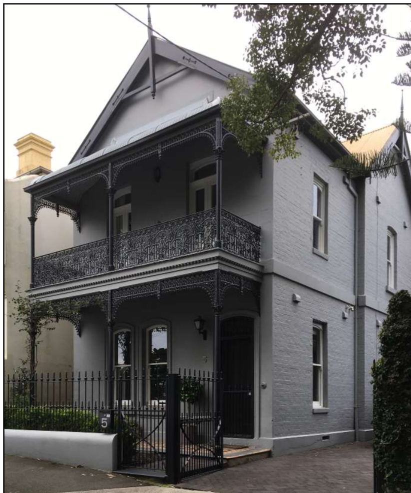
'Holroyd' (formerly 'Holyrood') Home of John Storey from 1913 to 1921 Pic Dale Keeling
