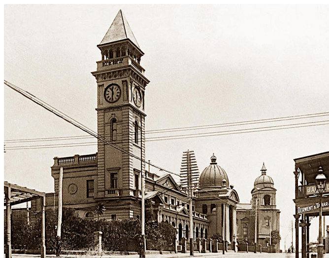
Image 13 (1014×786): The Balmain civic precinct c1907. 112 Note that the roof of the Post Office tower was clipped in the original photo and has been “photo-shopped” back in without its finial in this image-processed copy. Some overhead tram lines were also erased.
