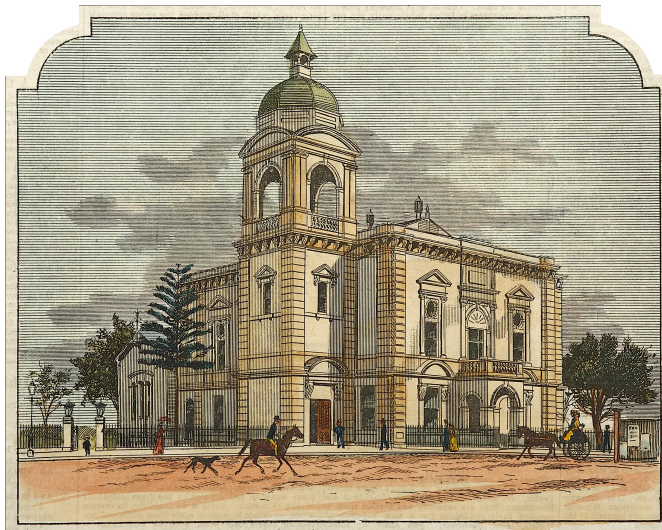
Image 1 (3548×2816): Hand-tinted newspaper clipping of a drawing produced for the opening of the Balmain Town Hall on 25 August 1888. 32,33 The cupola of the Victorian Free Classical building consisted of an octagonal dome supported by an arcaded storey and topped by a lantern.
